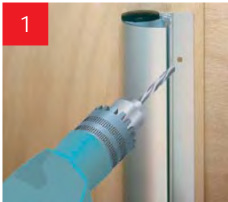
Drill pilot holes for A roller system housing
