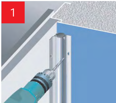
1 Drill pilot holes for A roller system housing
